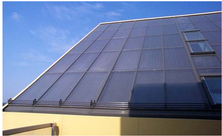
Figure 2: Solar roof with integrated windows and blind-elements without absorbers in temporarily shaded parts
