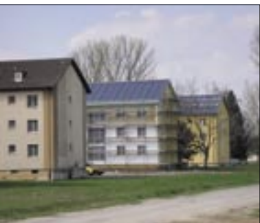
Fig. 11: Solar retrofitted and heat insulated apartment houses, converted from former military barracks buildings
