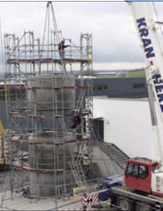
Fig. 1: Construction of the 100 m 3 buffer tank as diurnal storage for the central solar heating plant in Crailsheim, Germany
