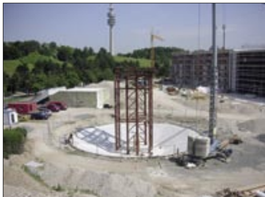
Fig. 7: Sequence of the construction of the tank thermal energy storage in Munich, 2006
